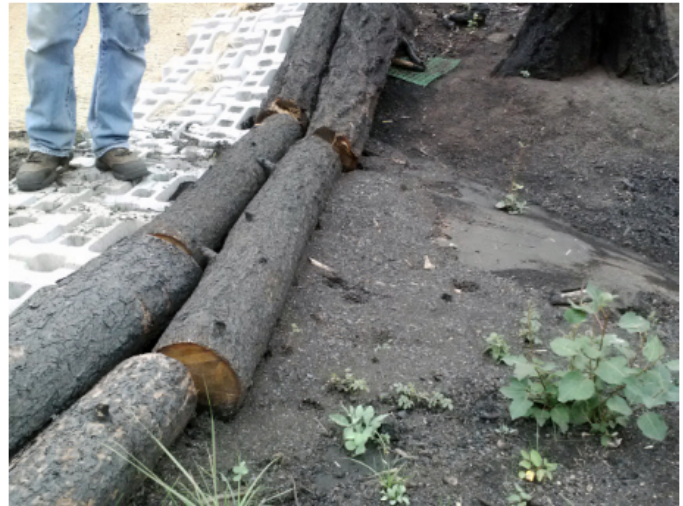
Figure 3. Sediment collected at the front of a log dam. Photo by B. Grotz.
